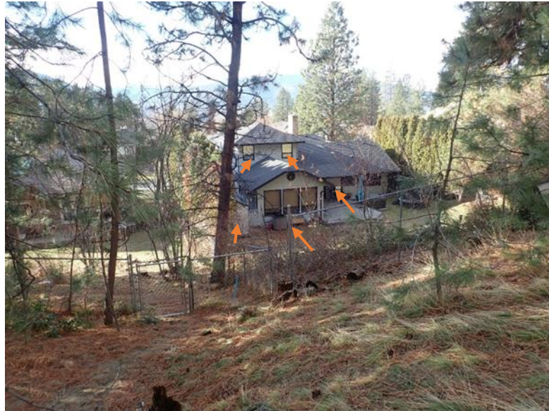
Figure 2. Areas of concern for fire ignitions and spread around a structure
