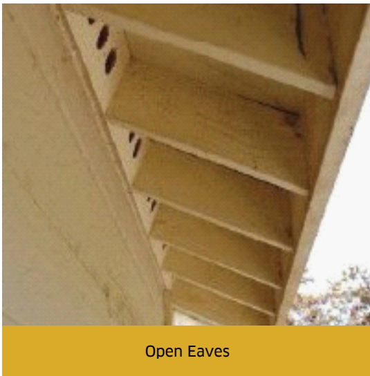
Figure 2. Open eaves with blocking and screening" (left) vs closed eaves using soffit with attic venting (right)
